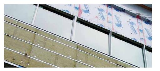
Exterior insulation installed in-between steel z girt cladding support attachment resulting in exterior insulation that is not continuous and does not meet energy codes (Source: Roxul, Inc.)
